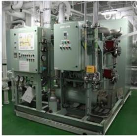
Figure 1.13 Membrane N<sub>2</sub> Generator System (Courtesy of Kashiwa Co., Ltd.)
