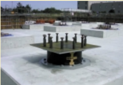
The laminated ferro-rubber shoe placed on a base block. These make the quake period longer and softer.
