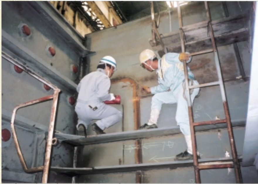
Close-up inspection of welding with SHI staff
