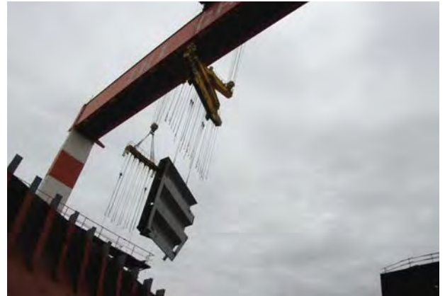
Block Construction at Aichi Works
