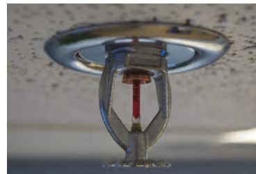
A fire sprinkler mounted on a ceiling (Wikipedia)
