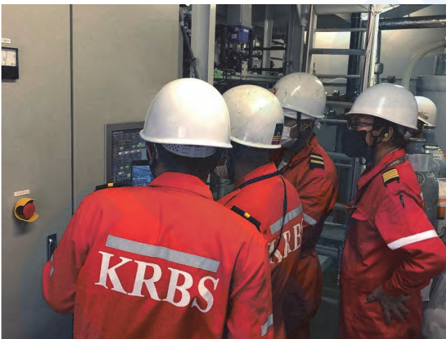
Fig. 7 Condition of demo plant operation
