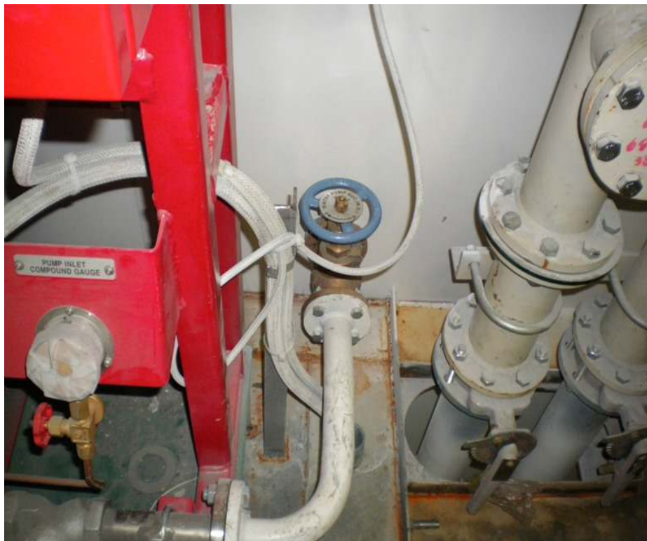
(1) Water supply valves to be always opened
