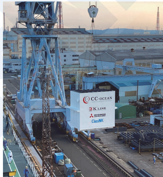
Fig. 4 Condition of demo plant room installation
