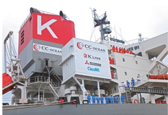
Fig. 6 Demo plant room after completion of installation on the ship
