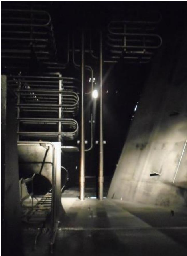
3. Tank sidewall and heating coils (From the top)
