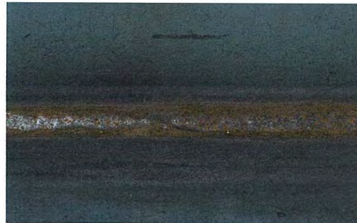
C1.3 Automatic fillet weld
