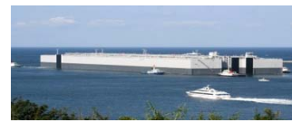
"KAMIGOTO" No.1 - 5 Total Capacity : 4,400,000 m 3
