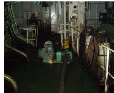
Oil is being pumped from the engine room
