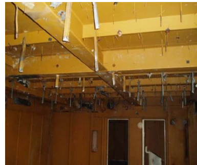
Pre-cleaned accommodation is ready for cutting
