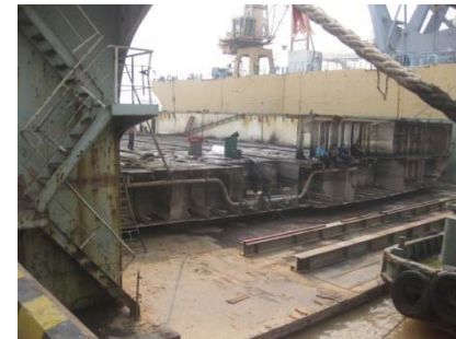
Floating dry-dock for final cutting
