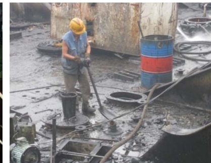
Cleaning of oily deposits
