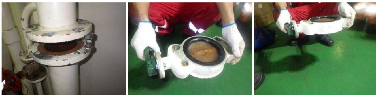
Photo Samples of Fire Main Isolation Valve Maintenance
