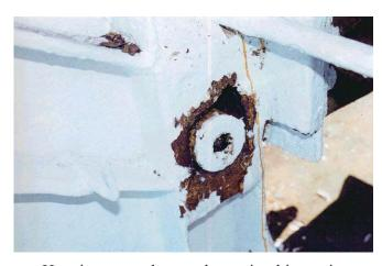
Housing wasted around carrying hinge pin
