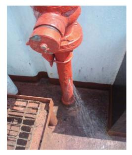
Leakage of fire line
