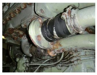
Inappropriate repairs by rubber patch on SW pipe for G/E
