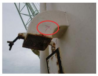
Hole with inappropriate repair with tapes
