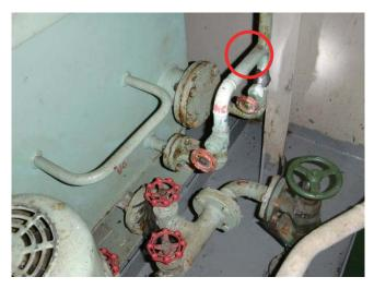
Inappropriate repairs by rubber patch and plastic putty
