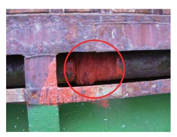
Inappropriate repair by cloth
