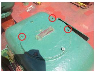
Missing bolts of air pipe head
