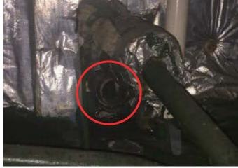
Partly missing A-60 class insulation
