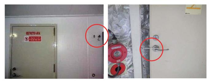
Unacceptable hold-back hook for door (required to be self-closing)!
