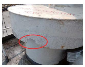
Wastage of the casing of ventilator
