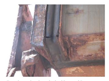
Deteriorated and cracked rubber packing
