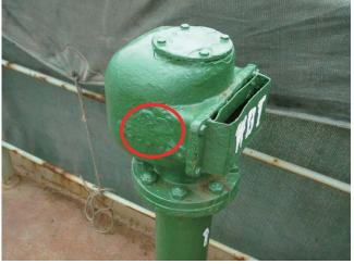
Inappropriate temporary repaired by putty
