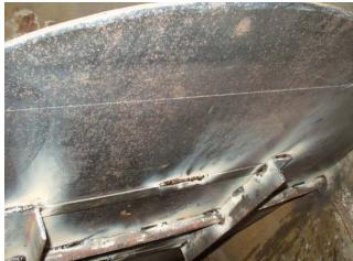
Wastage/Corrosion holes in fire damper flap
