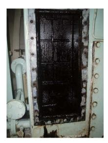
Oily inside of oil water separator
