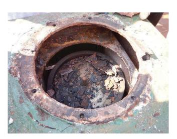
Excess Corrosion of inside of air pipe head
