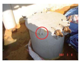
Missing nut and bracket with bolt
