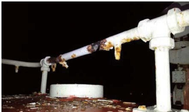
← Corrosion and Hole of water spray
