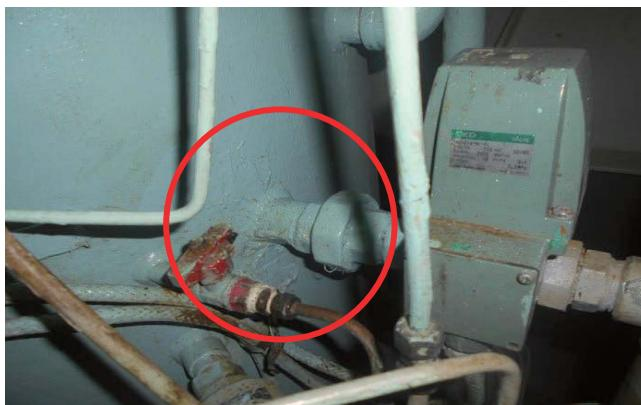
Illegal repair by patch with putty of Oily Water Separator
