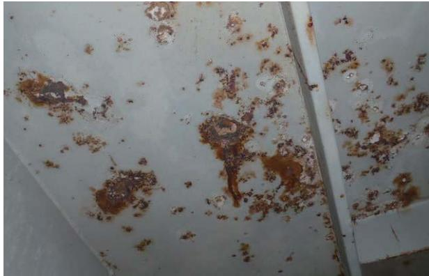
**Corrosion holes of strength deck**
