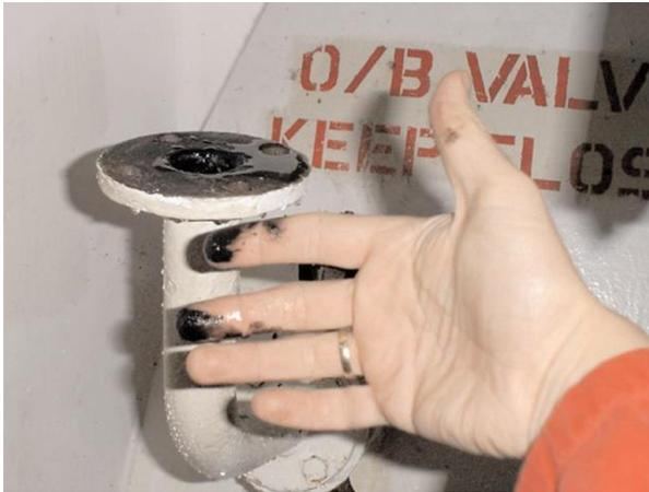
Oil contamination in overboard discharge line
