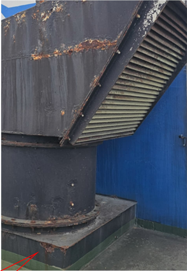
Corroded/Damaged ventilator
