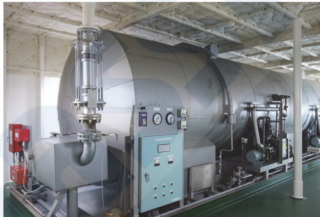
Fig. 5 Marine CO 2 fire-extinguishing system (−17°C/2.1MPa)
