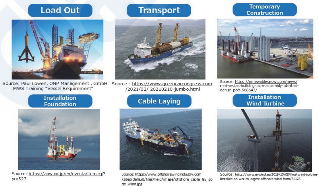
Fig. 4 Offshore wind farm construction processes
