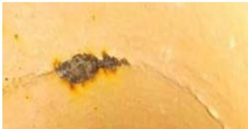
Picture 3 Paint peeled off at butt-welded parts of distance pieces
