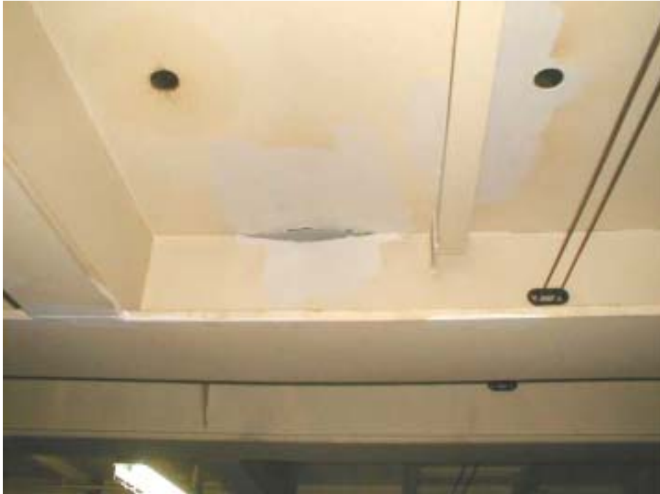
Photo 1. Detached tack welding between Web of Trans. and Deck plate
